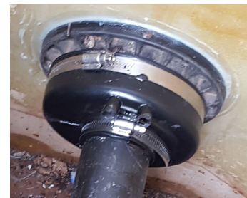
Example of Blueline Medium KFD Repaired
