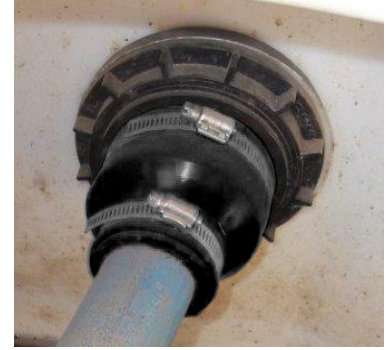
Example of OPW CS Medium Repaired
