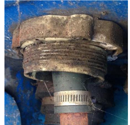
Example of TCI Direct Bury Fitting
