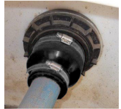
Example of OPW CS Medium Repaired
