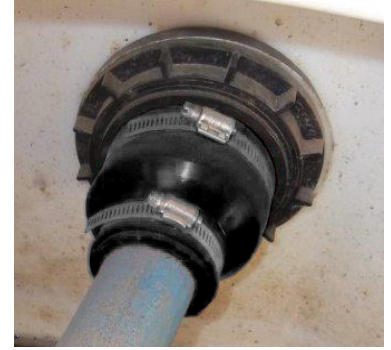
Example of OPW CS Medium Repaired
