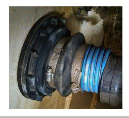
STEP 2 Re-seal Housing & Trim Ducting After pulling the existing product pipe out of the ducting, untighten the OPW fitting screw nut with a strap wrench, clean the area behind the nut, and dispense Icon PetrolSeal fitting gasket sealant completely around the threaded cuff where it enters the sump wall. Tighten the nut back completely.
