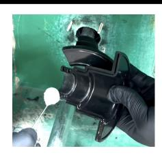
STEP 4 – Fitting Assembly After a 1-hour cure time, dispense gasket sealant onto the back of the Icon repair fitting or against the sump wall around the bolt pattern sufficient that when the fitting is compressed against the sump surface completely, it will provide a thin and complete coating between sump and fitting. Any excess should be wiped away at the end of the installation.
