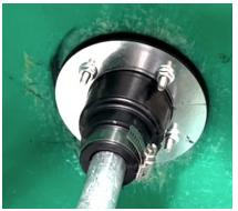
STEP 5 – Quality Check Assembly Make sure that all parts are seated/fitted properly and that all nuts and the band clamp are completely hand tightened (15-20 inch pounds) to assure a leak-tight compression seal. The repair is complete at this point and ready for hydrostatic or other testing at this point.
