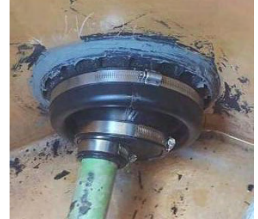
Example of Blueline Large KFD Repaired
