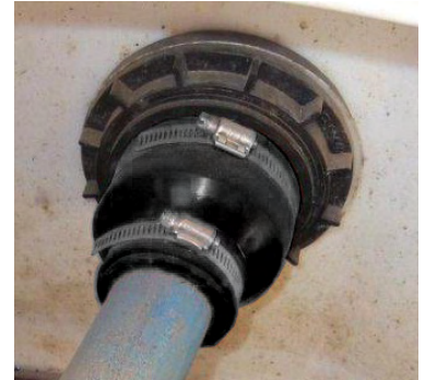
Example of OPW CS Medium Repaired
