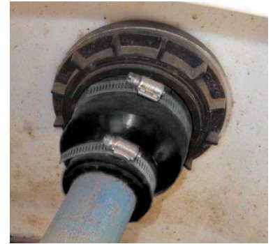
Example of OPW CS Medium Repaired
