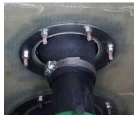
4-Bolt Nupi Fitting Example
