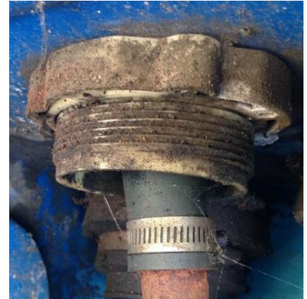
Example of TCI Direct Bury Fitting
