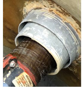
Example of Western Fiberglass Double-Wall Cuff Fitting
