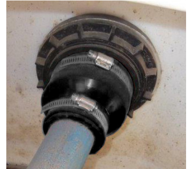
Example of OPW CS Medium Repaired
