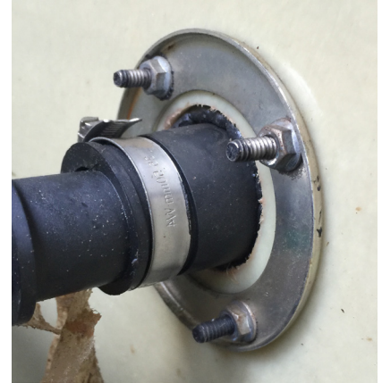
4-Bolt OPW Fitting Example
