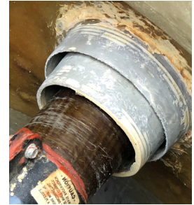
Example of Western Fiberglass Double-Wall Cuff Fitting
