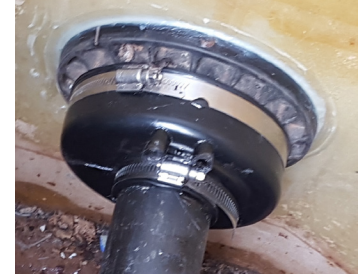
Example of Blueline Medium KFD Repaired
