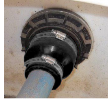
Example of OPW CS Medium Repaired
