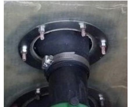
4-Bolt Nupi Fitting Example
