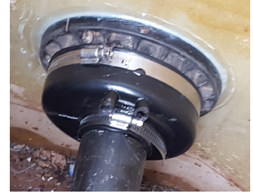
Example of Blueline Medium KFD Repaired
