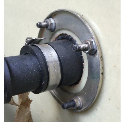
4-Bolt OPW Fitting Example
