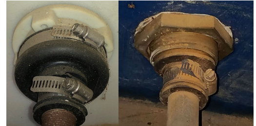
Examples of TCI Conduit Fittings
