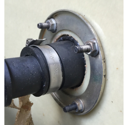
4-Bolt OPW Fitting Example
