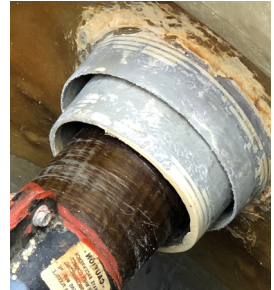
Example of Western Fiberglass Double-Wall Cuff Fitting
