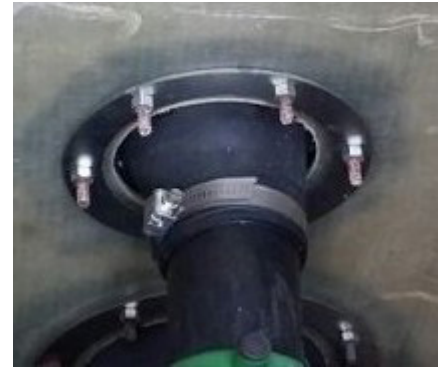
4-Bolt Nupi Fitting Example
