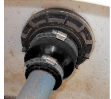
Example of OPW CS Medium Repaired
