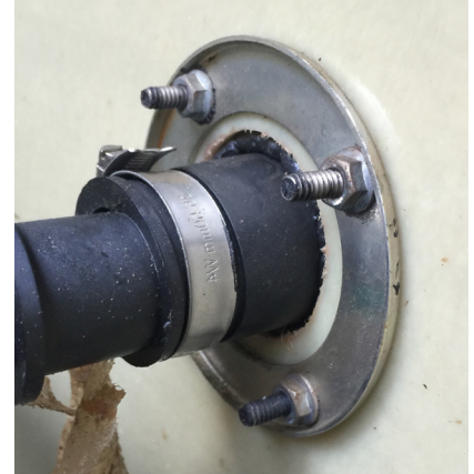
4-Bolt OPW Fitting Example
