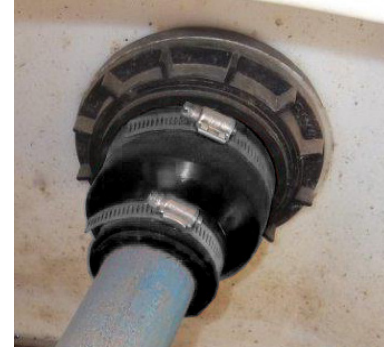
Example of OPW CS Medium Repaired
