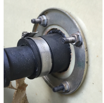
4-Bolt OPW Fitting Example
