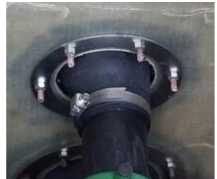
4-Bolt Nupi Fitting Example
