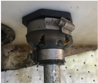
Example of OPW Conduit Fittings
