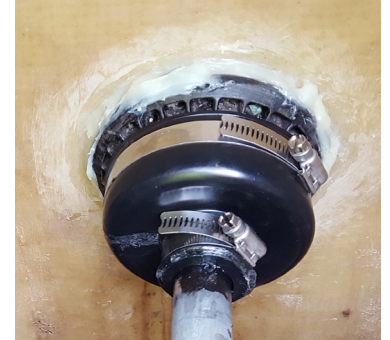
Example of Blueline Small KFD Repaired
