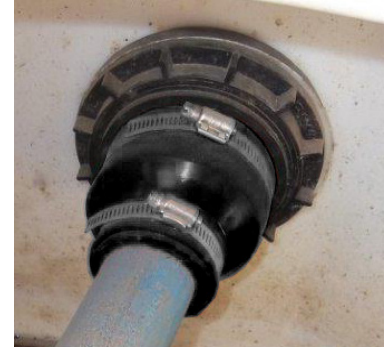
Example of OPW CS Medium Repaired
