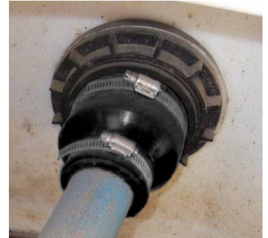
Example of OPW CS Medium Repaired
