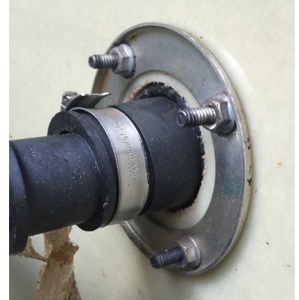
4-Bolt OPW Fitting Example
