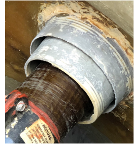
Example of Western Fiberglass Double-Wall Cuff Fitting
