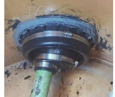
Example of Blueline Large KFD Repaired
