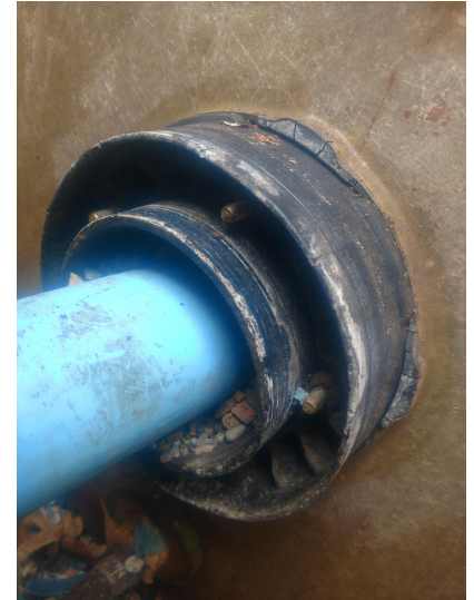
Blueline K2 Fitting w/ Degraded Boots
